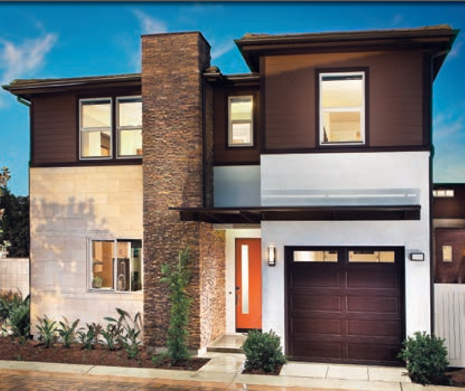
(Left Wall) French Limestone with 4" Chiseled Limestone Band - Country Beige (Center Column) Mountain Strip Stone - Chablis
